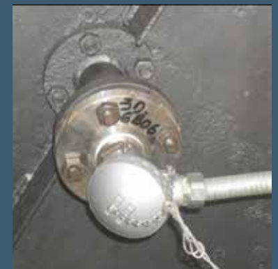
IMAGE ABOVE: Example of TSTC entry into furnace firebox.
